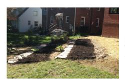
This is a vegetable garden which we created on contour and directed the roof runoff into a perforated pipe and buried the pipe in gravel. All of the water from the roof infiltrates into the soil and waters the vegetable beds.
