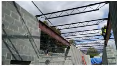
New roof joists at Area B (New pentagon wing)
