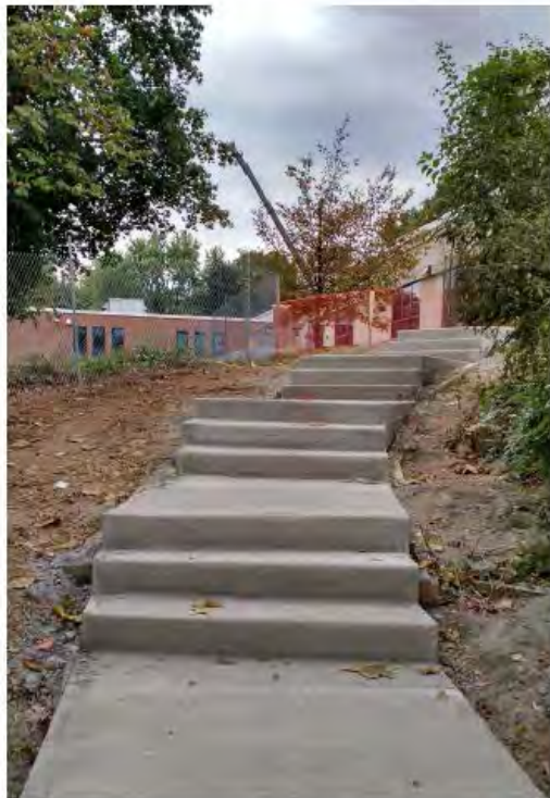
New concrete steps to the Relocatables
