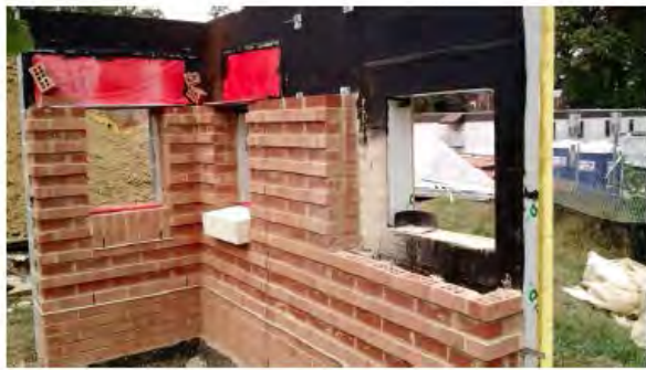
Mock Up wall in progress
