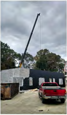
Roof joist installation at Area B
