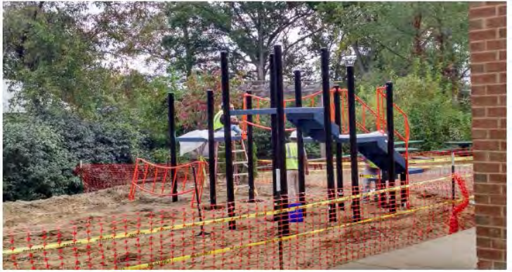
Temporary Playground installation
