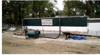
Temporary boilers onsite
