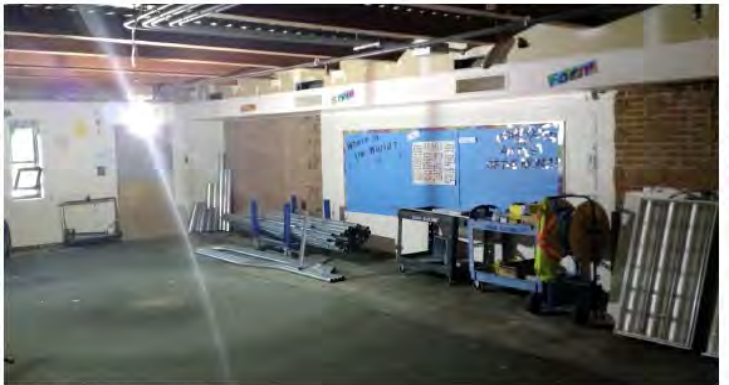
Old music room gone, new work under construction
