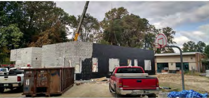
Area B construction
